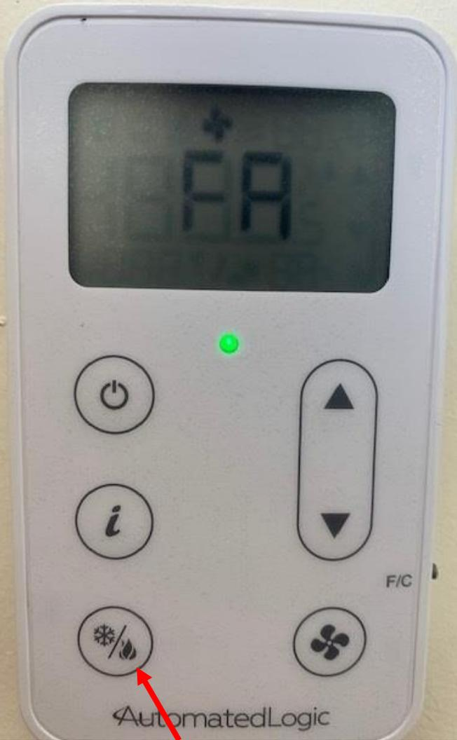
If the occupancy light is green (either from the occupancy sensor, or manually through the push button), then you may use the cool button. The first push will have the words "fan only" scroll across the screen.
